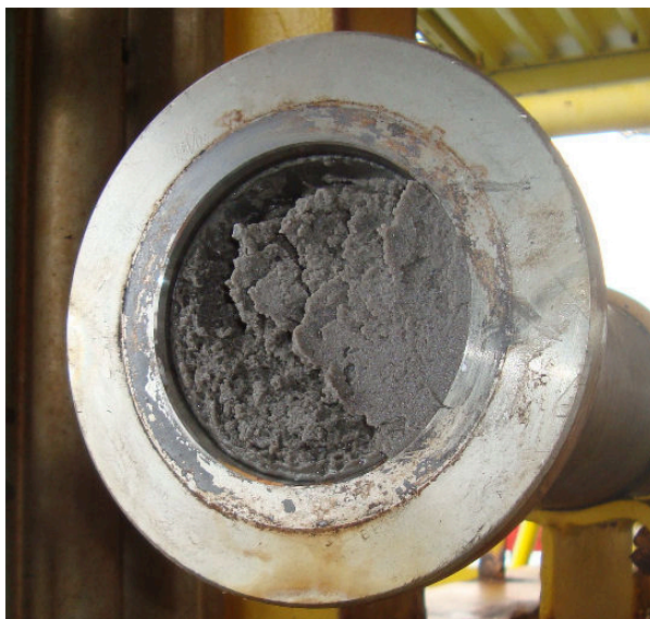
Example of too much sand being produced
